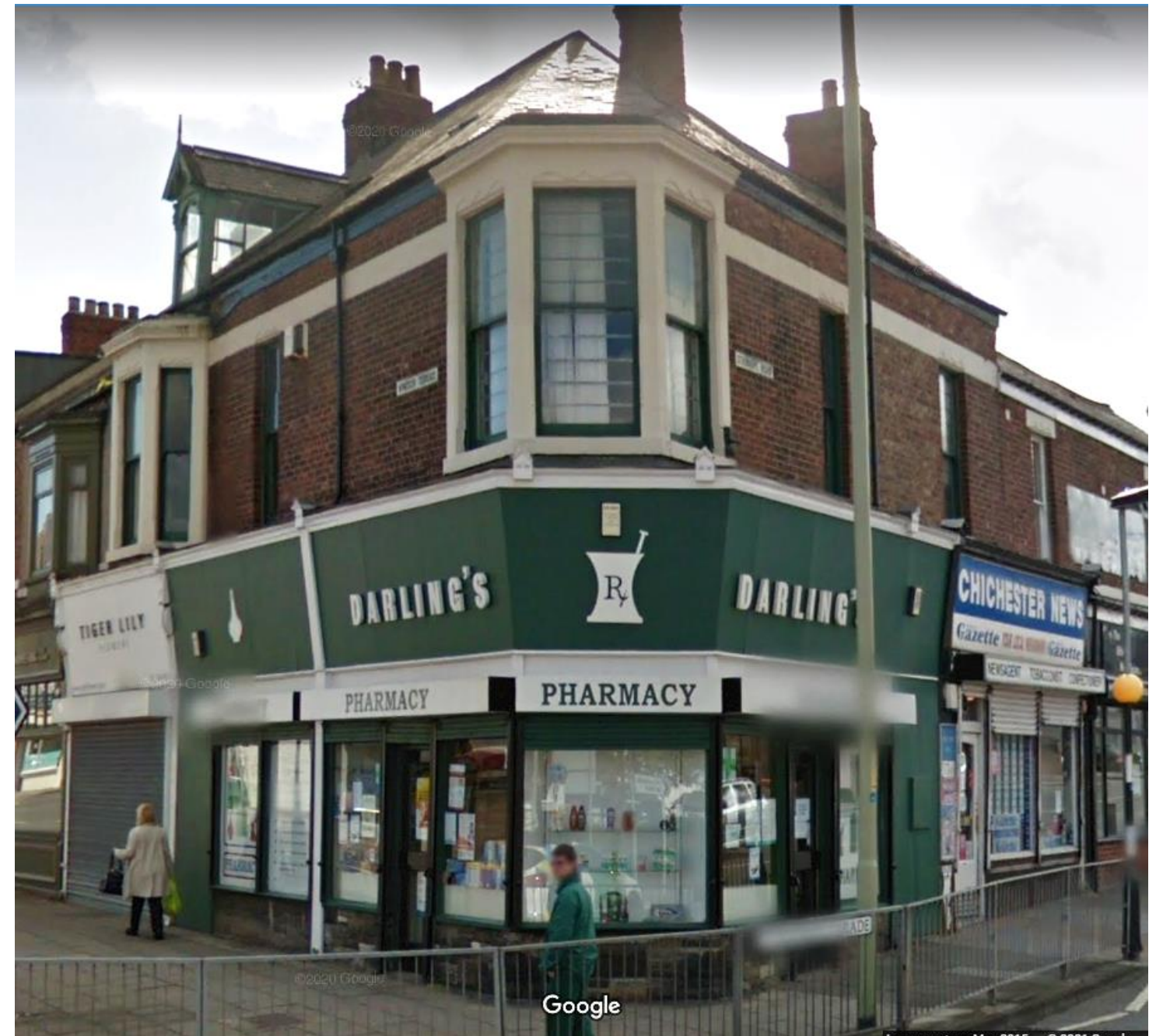
Fig. 2 – The premises & adjoining units prior to works (Image: Google Streetview)
